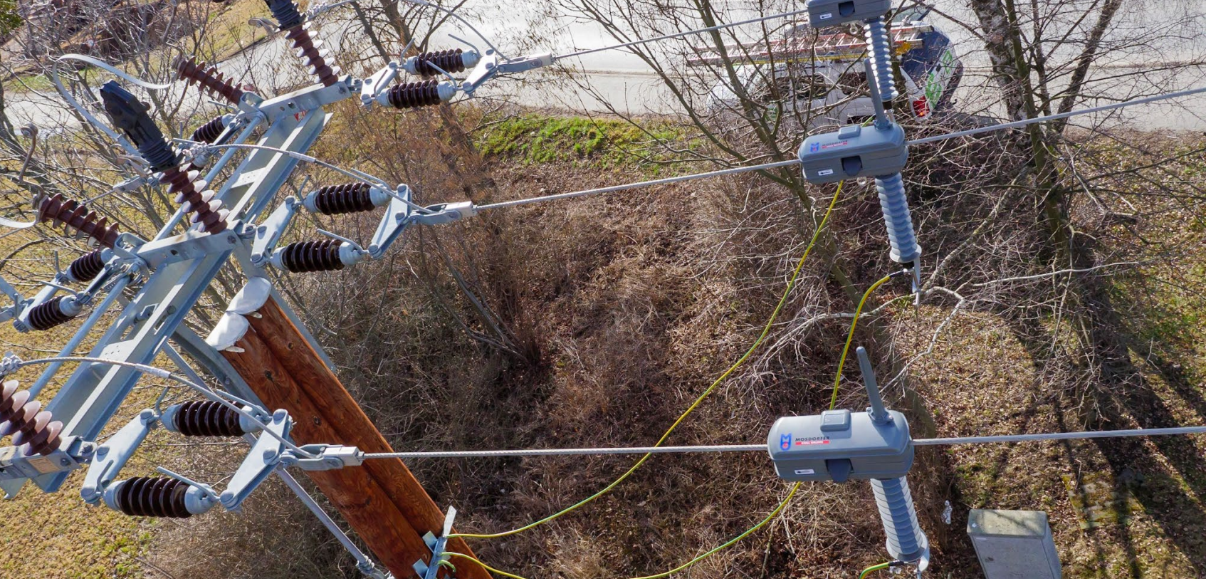
Aclara sensors for power line management between 1 and 65 kV
