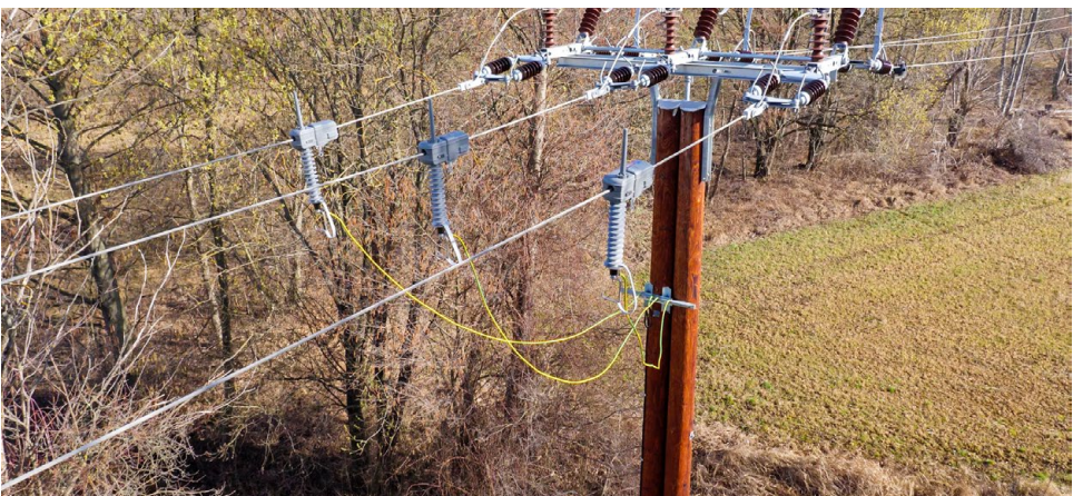
The sensors deliver important readings at 15-minute intervals, measuring the cable temperature, voltage and phase angle.
