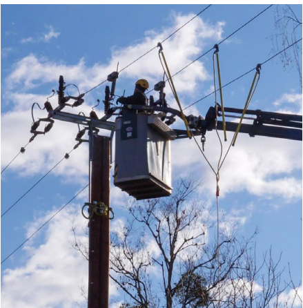
Installation of the three Aclara sensors took no more than half an hour, using a hydraulic platform.
