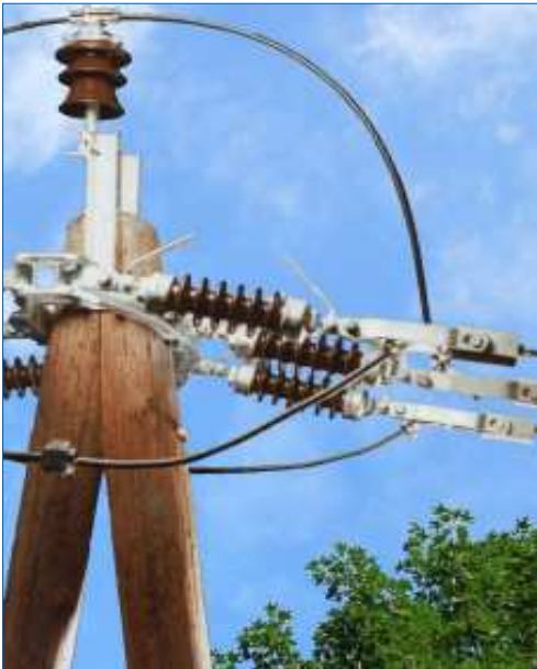
A-shaped tension tower
