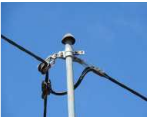
Roof pole with Roller suspension clamp
