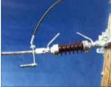
Dead end string with compression clamp
