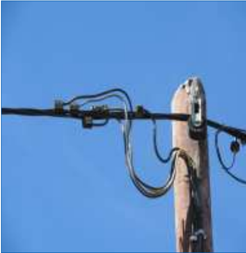
Piercing connectors on a suspension pole
