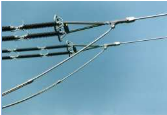
Loop guidance of a tension string
