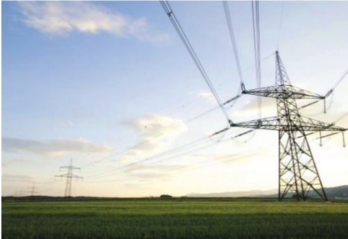
400 kV corner mast with OPGW earthwire
